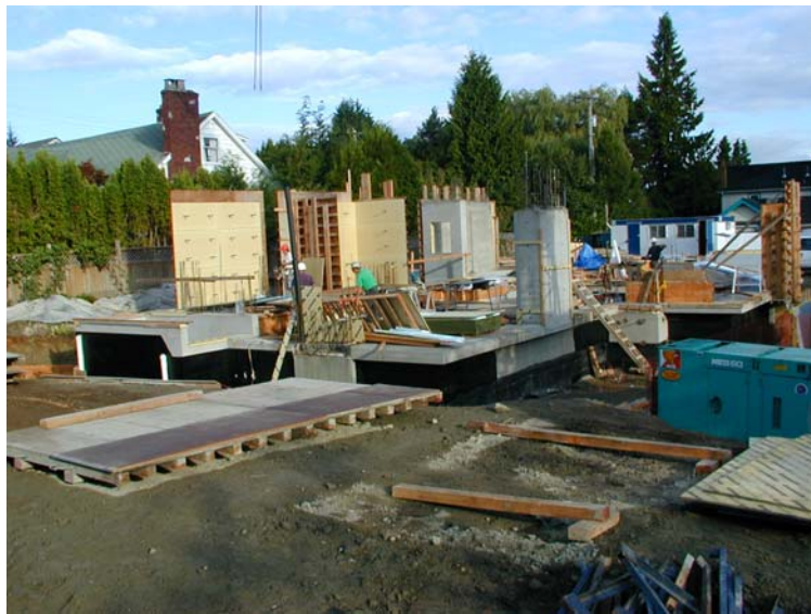
Figure B-4: View during Ground Floor Construction
