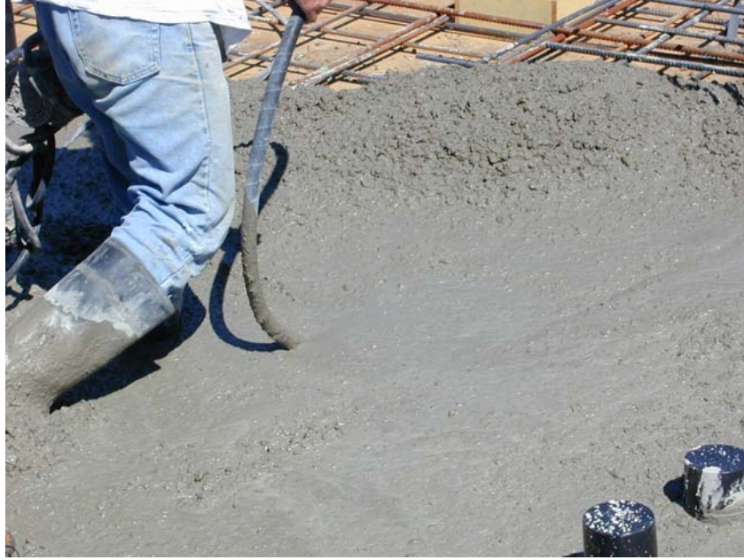
Figure 6: Close-up during Vibration
