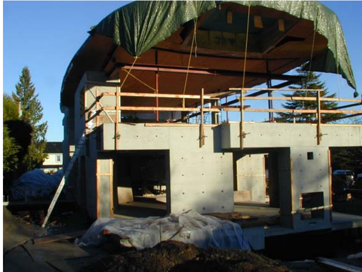
Figure B-1: South Wall
